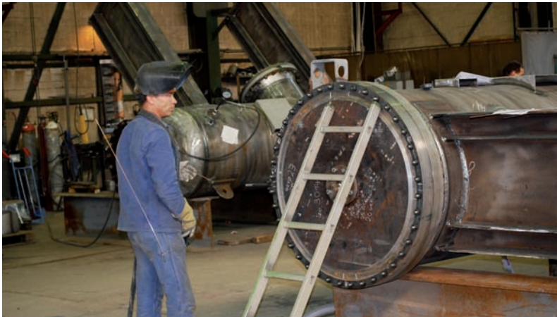
Fig. 8b: manufacturing of a Krone KAF 24" Car- bon Steel Unit
