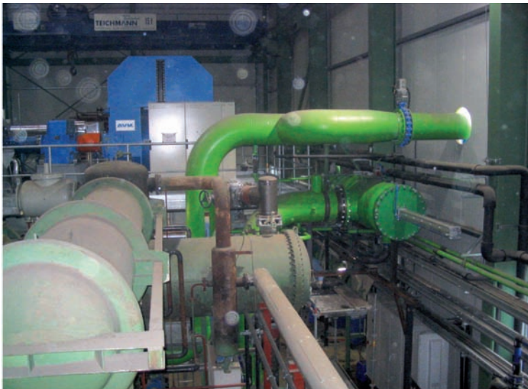
Fig. 8a: Filter with a nominal connection diameter of 600 mm in the cooling loop of a biomass power plant.
