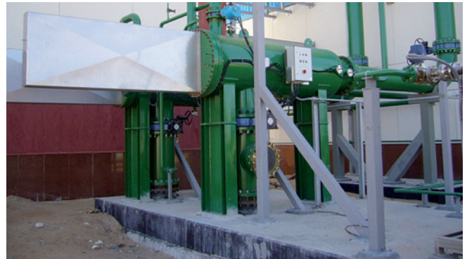
24"/DN 600 KAF® Filter – Seawater cooling
