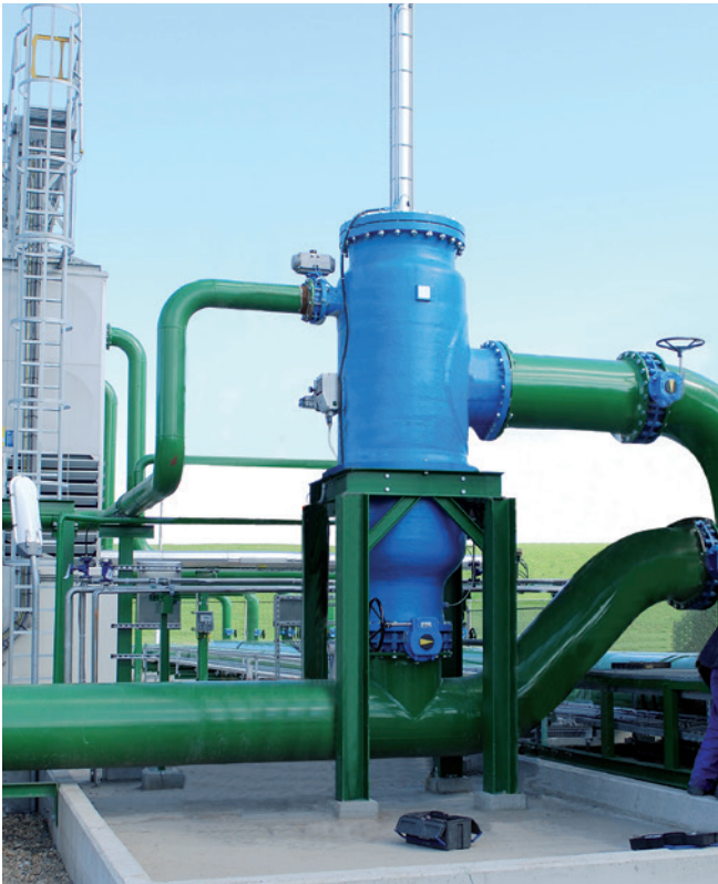
24"/DN 600 KAF® Filter – Bioethanol plant
